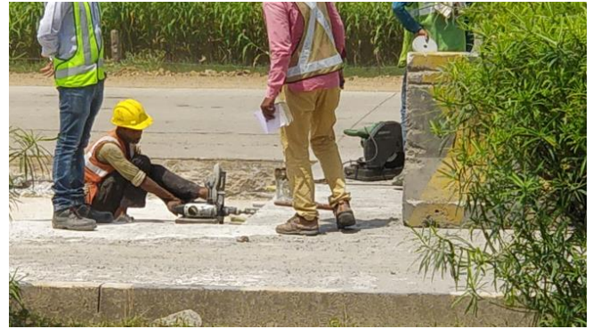
Repair work on existing four loan concrete road
